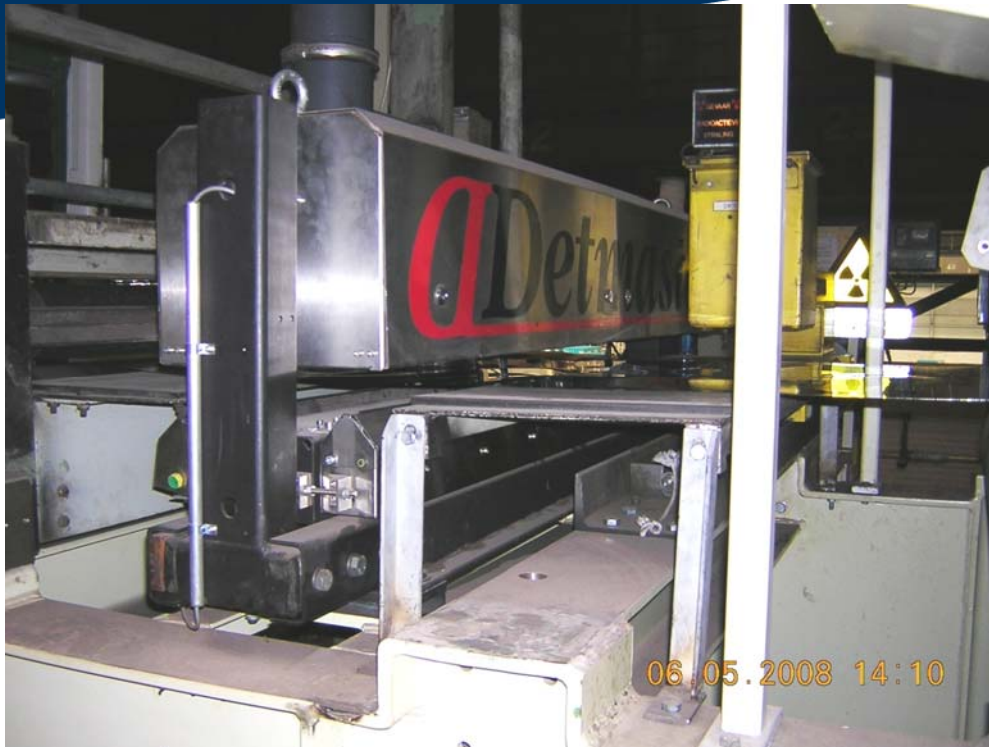
Picture 1 Detmaster 1400 MPH pinhole detection system installed on Inspection Line No. 12
